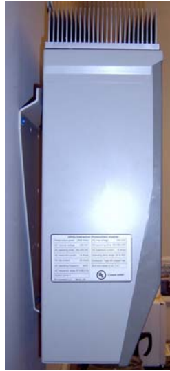
Figure 2: Inverter with mounting bracket in place
